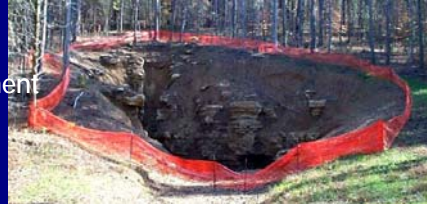
Left Abutment Sinkhole – Center Hill Dam
