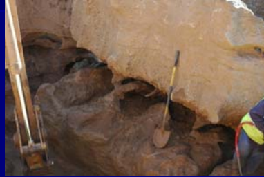
Stratigraphically controlled Karst with no connection to base of dam
