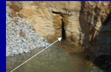
Open flowing 20 to 30 gpm under low head
