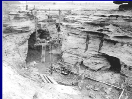
Caves along cutoff trench - Wolf Creek Dam
